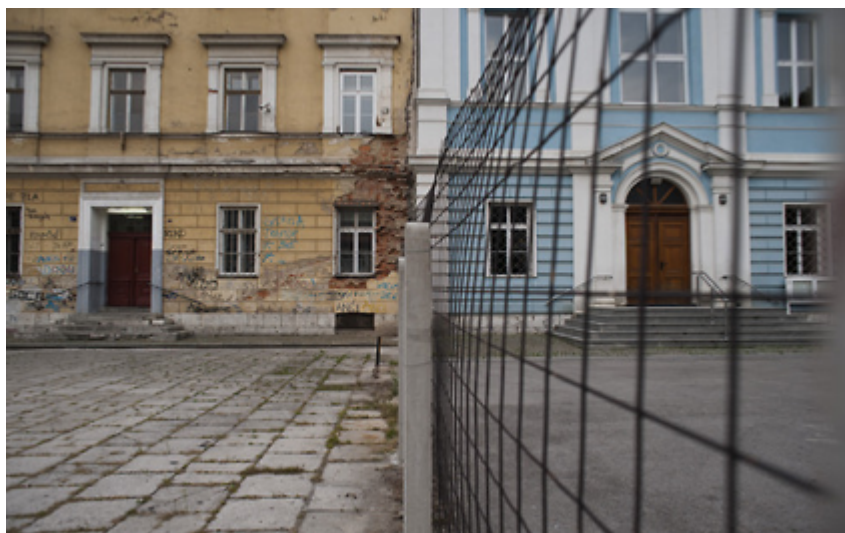
Fig. 3: The fence between the two parts of the divided gymnasium in Travnik
